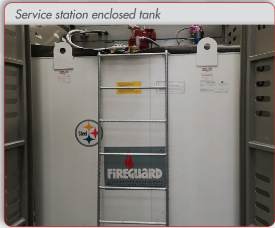
Small Service station system for motor spirit
